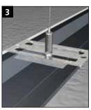
Push the running rails into the carrier profiles and align to the position marked ex works. Re-adjust the suspension height by applying pressure to the cable holder. To do this, raise the ceiling element on one side by approx. 30 - 40 cm and pull the wire ends diagonally to the carrier profile.
